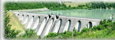
Val Grosina Dam 1958-1959
