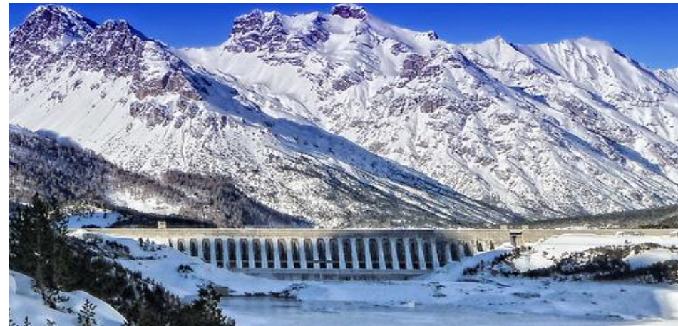
San Giacomo dam after new constructions
