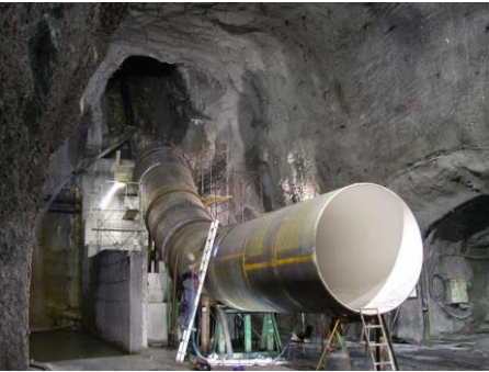
• Ø=2100 - L=1000 m new Penstock
