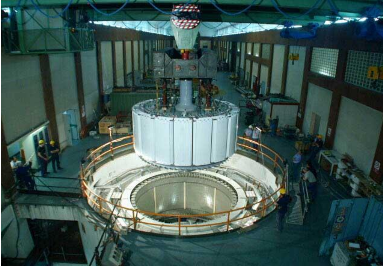
Installation of the 4th Generation Unit - 110 MW
