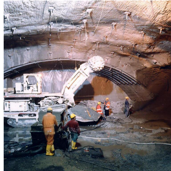
Excavation by roadheader
