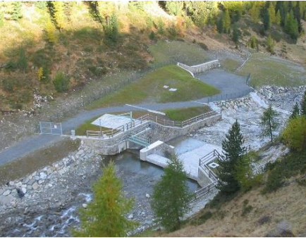
7 new water intakes
