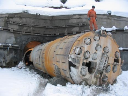
20 km water tunnel
