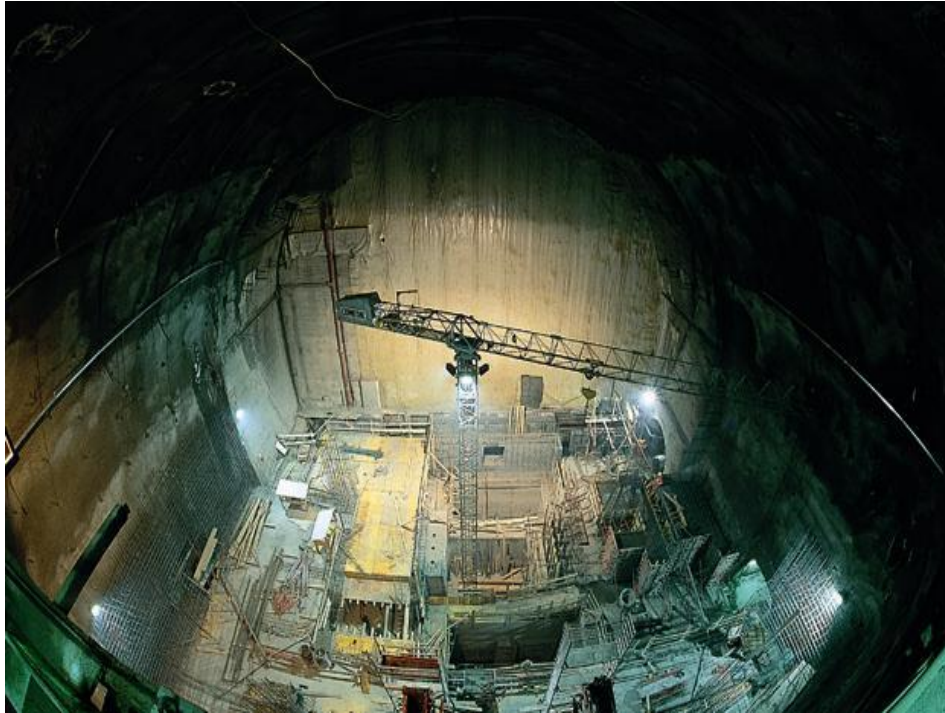
Extension of powerhouse in cavern
